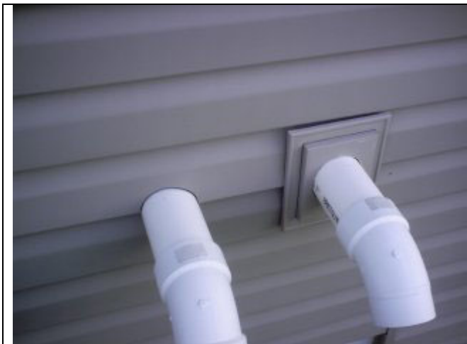
Seal around pipes.
