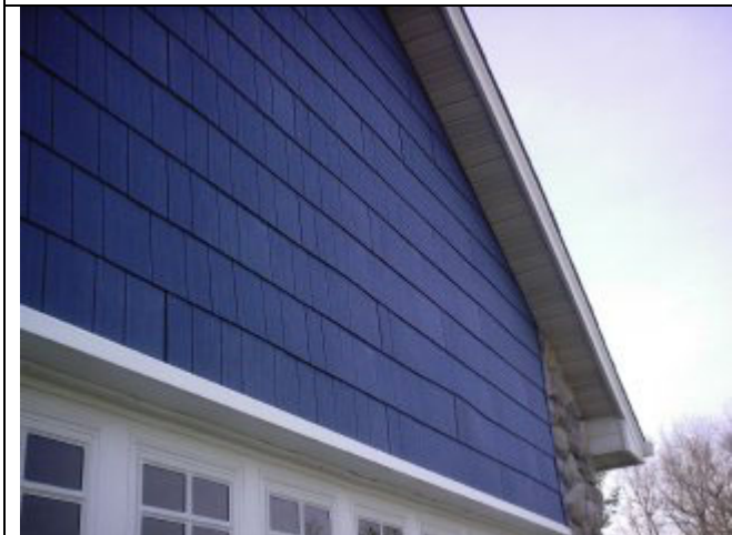
Warped plastic shingles.
