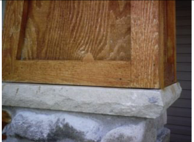
Seal areas around wood posts.
