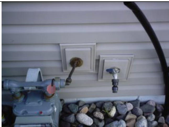
Seal around pipes.
